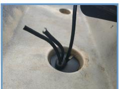
Now pull tight and position the cover into the hole. Make sure the
